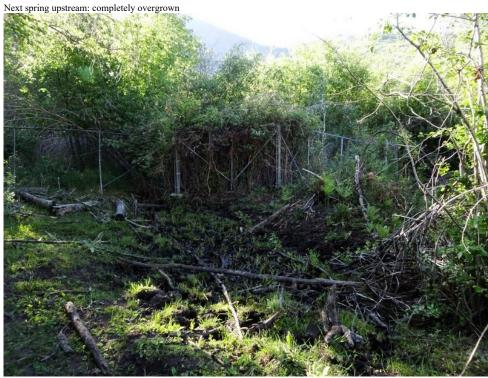
The gate cannot be opened due to the overgrowth at this Bell Creek spring. The spring box can no longer be maintained. A meter is needed here.
